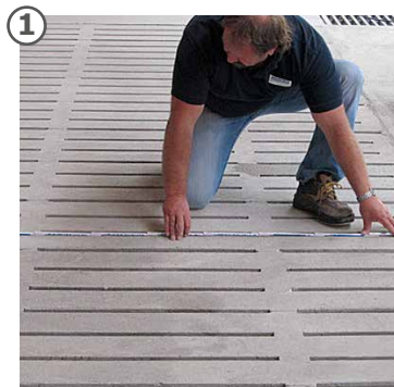
slatted floor is measured
