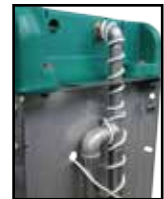
Heated option, connection to water circuit with frost protection heating cable wrapped around the valve
