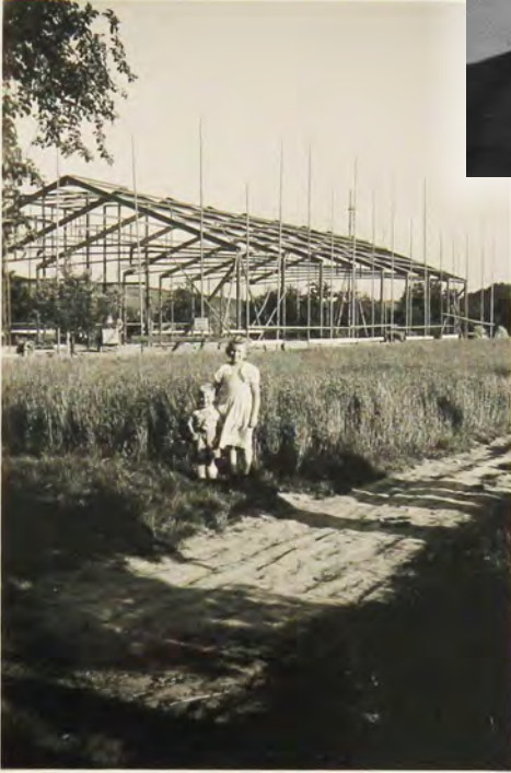
Frank Haiges with his cousin Inge in front of the new foundry building in Kirchheim am Neckar
